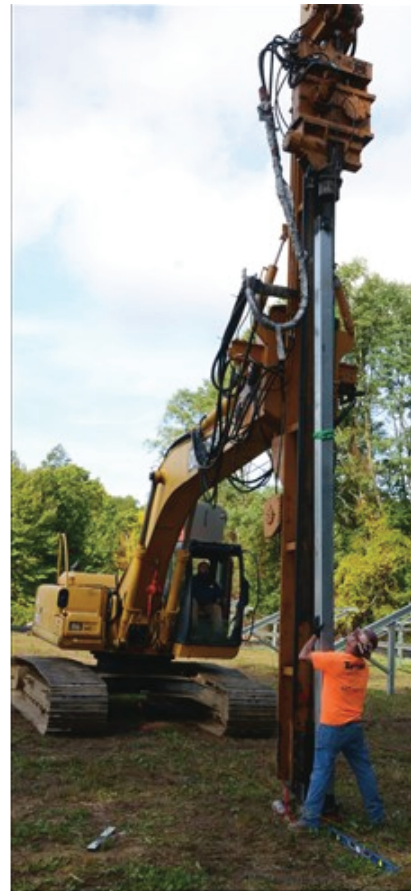
A driver, time-wise, for the construction schedule of the Mt. Tom solar project was a Commonwealth of Massachusetts incentive program. ENGIE North America wanted to ensure that the project schedule met the incentive deadlines, as well as the timeframe set by Holyoke Gas & Electric.
